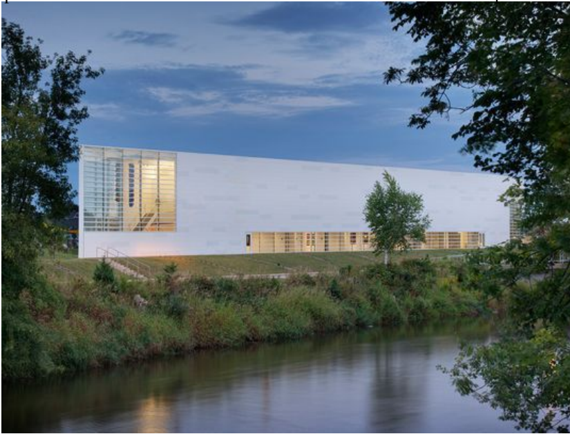
HGA Architects and Engineers designed the Museum of Wisconsin Art in West Bend. It overlooks the Milwaukee River. (Photo: Darris Lee Harris)
